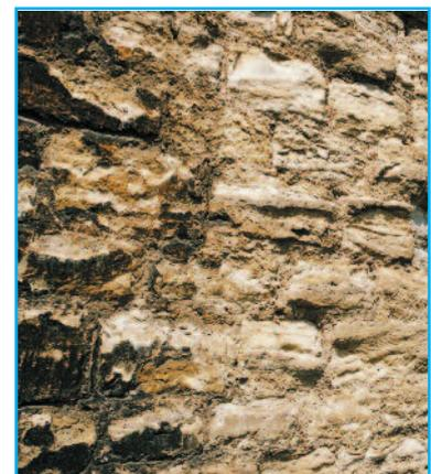
Image depicts a typical stone wall damaged by contaminants.
